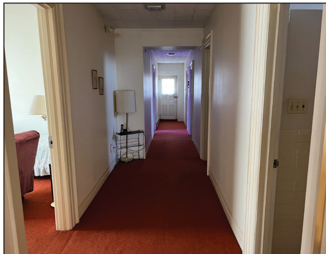
The Cathedral Convent building has three floors, this is the top floor of the building, which will soon receive new carpeting, paint and other necessary updates. (Photo/Eric Deabill)
