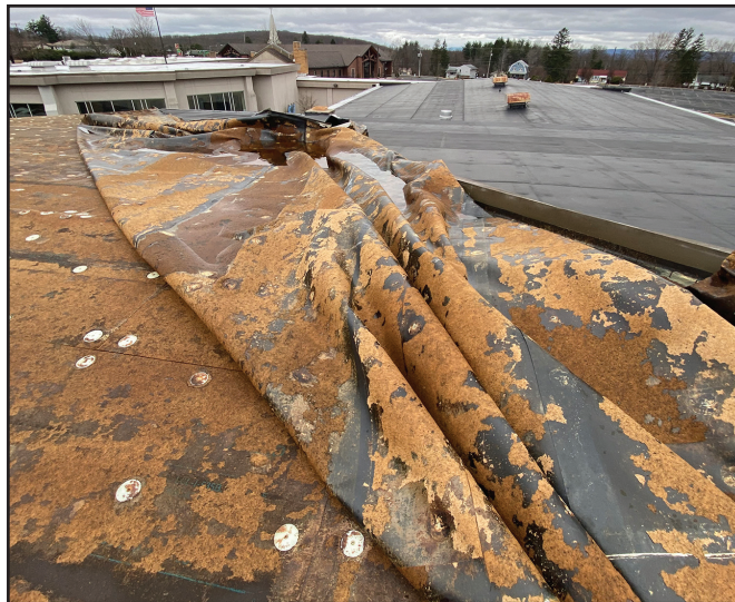
During a major wind storm in March 2025, the roof of Saint Jude School in Mountain Top was severely damaged. This roof was among five major roof replacements completed this summer at Catholic schools.
