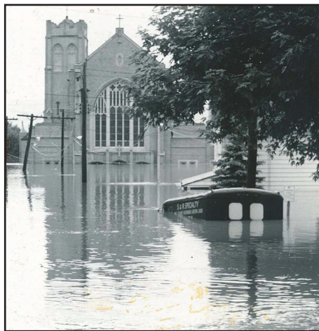
Flood waters from the Susquehanna River inundated Saint Aloysius Church in July 1972. This photo was taken when water was nearly to the top of the church doors.
